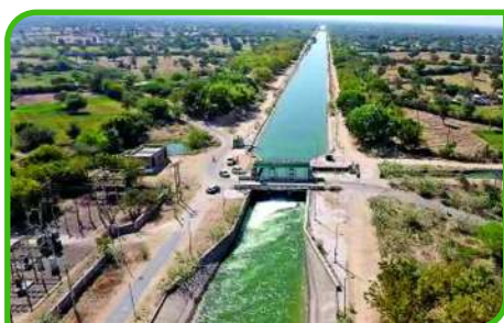
World's Largest Lined Irrigation Canal Narmada Canal.
